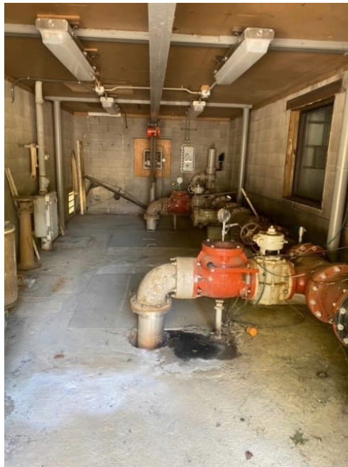
Figure 2-4. Main Lift Station Upper Floor
